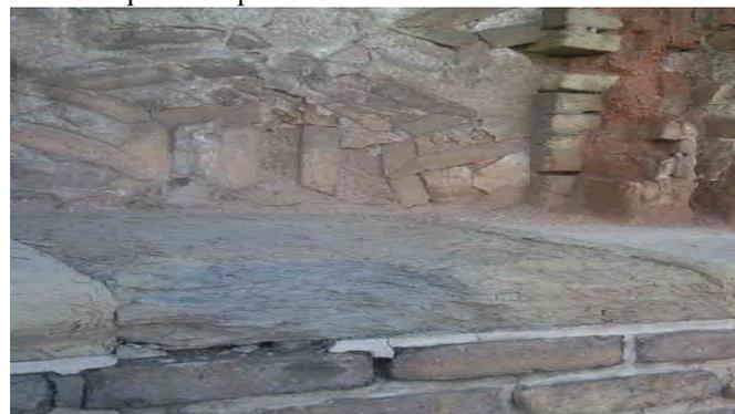
Fig. 3 Decomposition of stones due to acid rains
