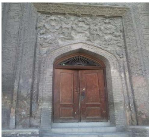
Fig. 4 Moisture along with fluctuations in temperature can lead to disintegration of the façade (plasterwork) in cold regions (Alavian dome, Hamadan, Iran)
